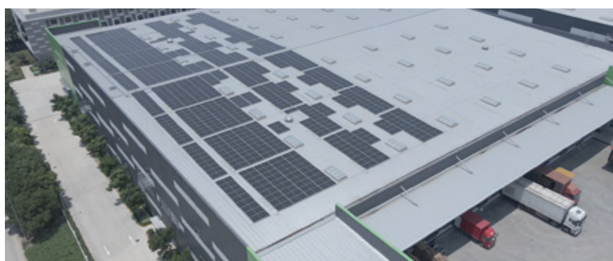
Solar photovoltaic system in Forest Shanghai Fengxian Logistics Park
