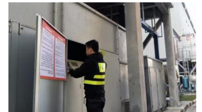
Refrigeration unit inspection
