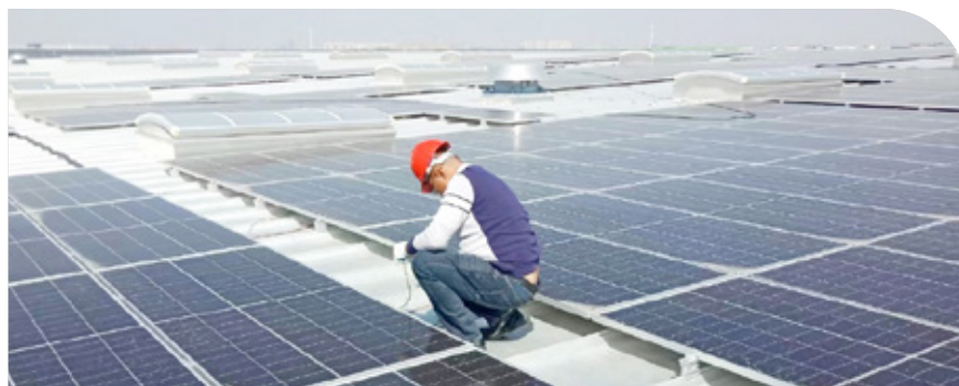
Rooftop solar photovoltaic system under inspection
