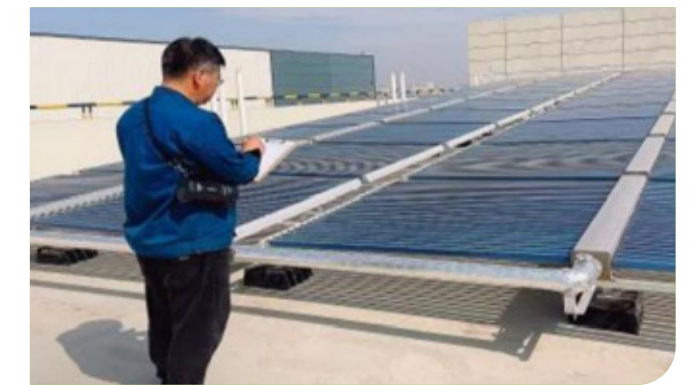
Solar energy system inspection
