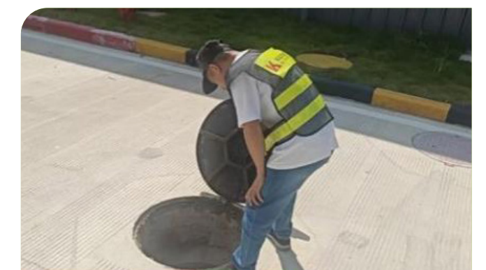
Drainage system inspection
