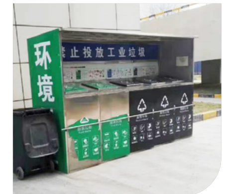
Waste recycling facilities in the logistic industrial distribution warehouses
