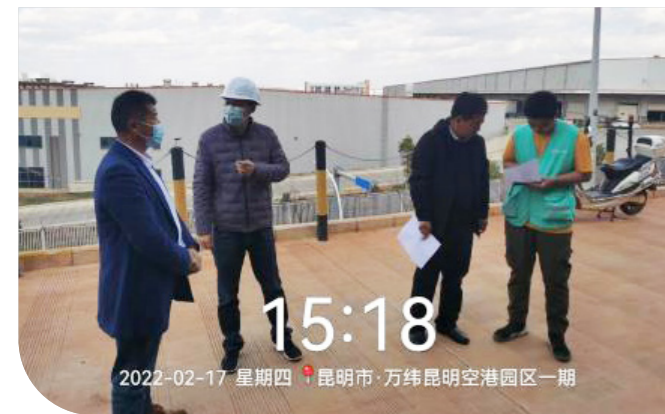
Onsite safety inspection
