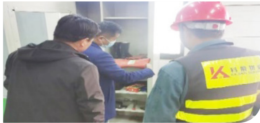
Onsite safety inspection
