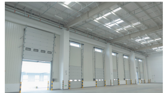
Maximize the use of natural light in our logistic industrial distribution warehouses
