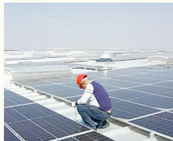
Rooftop solar photovoltaic system under inspection
